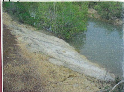
Figure 29. Nov 05. Rain-filled Pond 3 showing moat partially filled (note red road base soil on top of dike).
