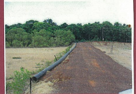
Figure 31. Nov 05. Delivery seawater Pipe to be connected to intake pump.
