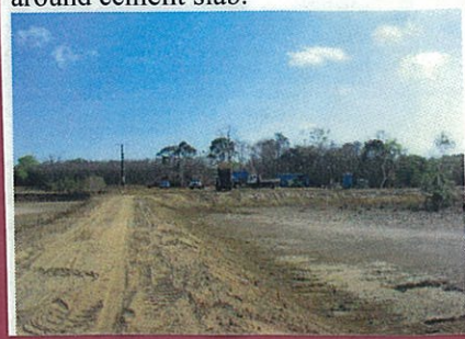
Figure 18. Oct 05. NE view of base camp showing work vehicles parked around cement slab.
