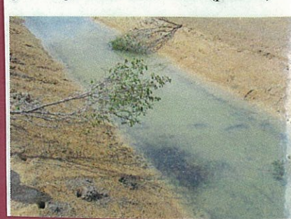
Figure 21. Oct 05. Crab shelters made from up-rooted mangroves growing inside dike walls (pond 3).
