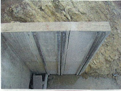
Figure 32. Nov 05. Monk walls cut for inserting sluice boards.
