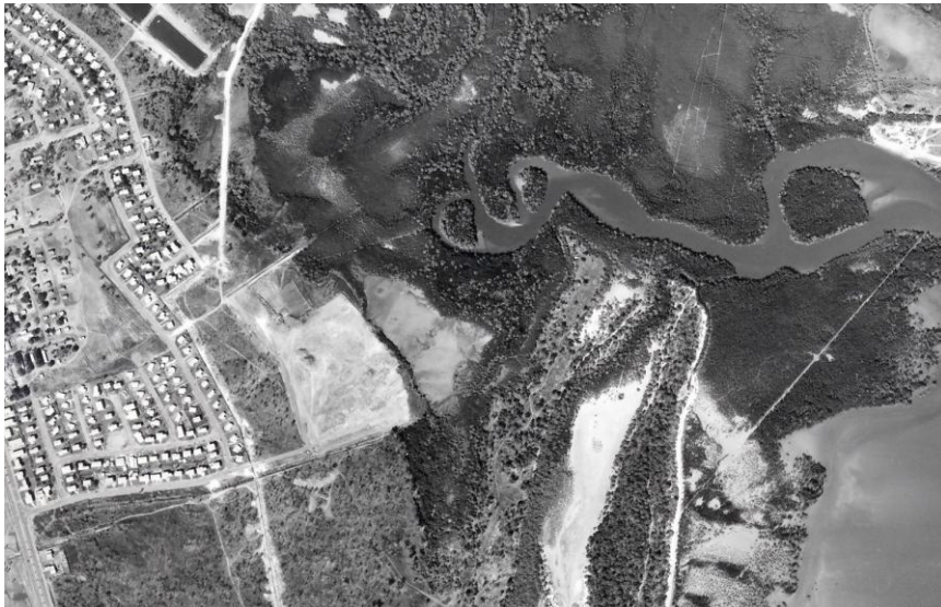
Figure 1 (above): The Ludmilla dump site in the 1974 before it was extended further into the mangroves after Cyclone Tracy.
