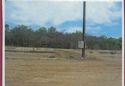
Figure 16. Oct 05. Second power pole with a junction box between settlement ponds 1 and 2.
