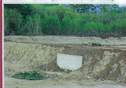
Figure 25. Nov 05. Concrete collar to support drains between settlement Ponds 1 and 2 (note red road base).
