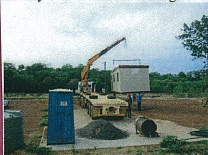
Figure 27. Nov 05. Demountable delivered to base camp and positioned directly over foundation footings.
