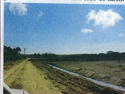
Figure 19. Oct 05. NE view from pond 3 with seawater seepage from pond monk on the creek side of farm.
