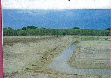
Figure 29. Nov 05. Rain-filled Pond 3 showing moat partially filled (note red road base soil on top of dike).
