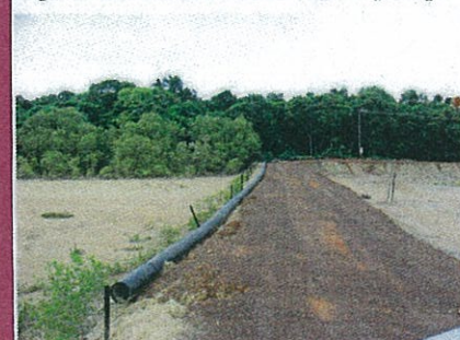
Figure 31. Nov 05. Delivery seawater Pipe to be connected to intake pump.
