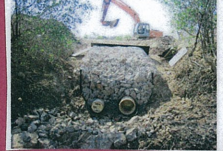
Figure 8. Sept 05. Construction of Drain/Intake for Pond 1 on creek side.
