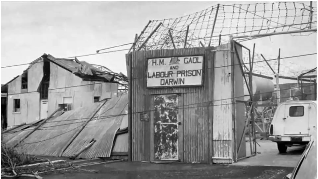
Fannie Bay Gaol on Christmas Day, 1974, following Cyclone Tracy. Short-term prisoners like Fred Fogarty were released after the cyclone severely damaged the prison.
