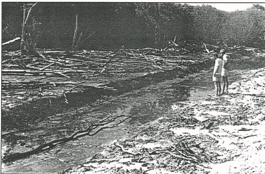
Photograph Eighteen: The Mosquito Drains. This drain lies along a tidal creek line which runs parallel to Ludmilla Bay from Coconut Grove to Ludmilla Creek – the dead mangroves may be the result of Cyclone Tracy, but regeneration has been retarded by the impedance of tidal flushing due to a siltage block downstream and the restriction of fresh water input from the upper reaches of the creek (Henderson 1984)
