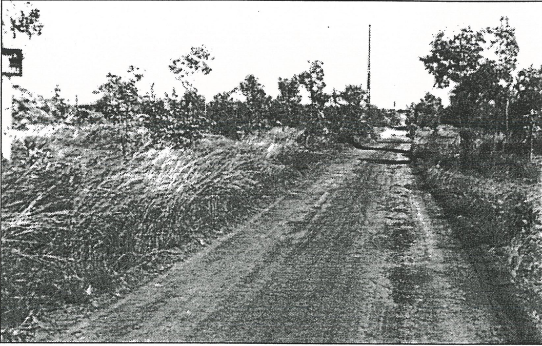
Photograph Eleven: The Coconut Grove road before Dick Ward Drive was constructed – note the Gwalwa Daraniki sign to the left (Northern Territory Archives, WB Day Collection NTRS 75 Photo 79)
